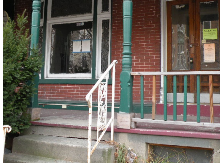
Concrete porch slab in 2012. (HARB files)
