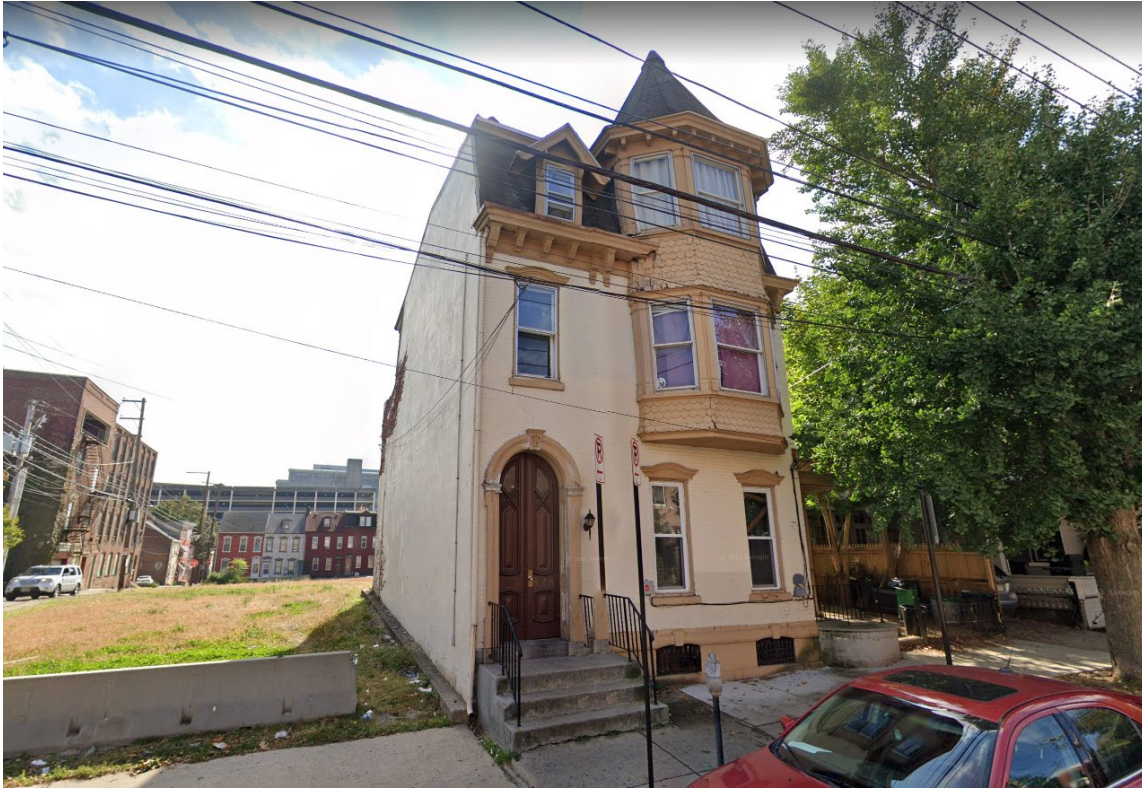
Front façade of 828-30 W. Turner Street, 2021. (Google StreetView)
