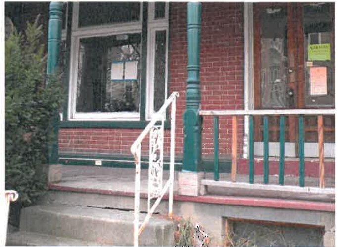
Concrete porch slab in 2022. (HARB files)
