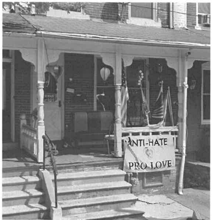
Detail of porch, 2021. (Google StreetView)
