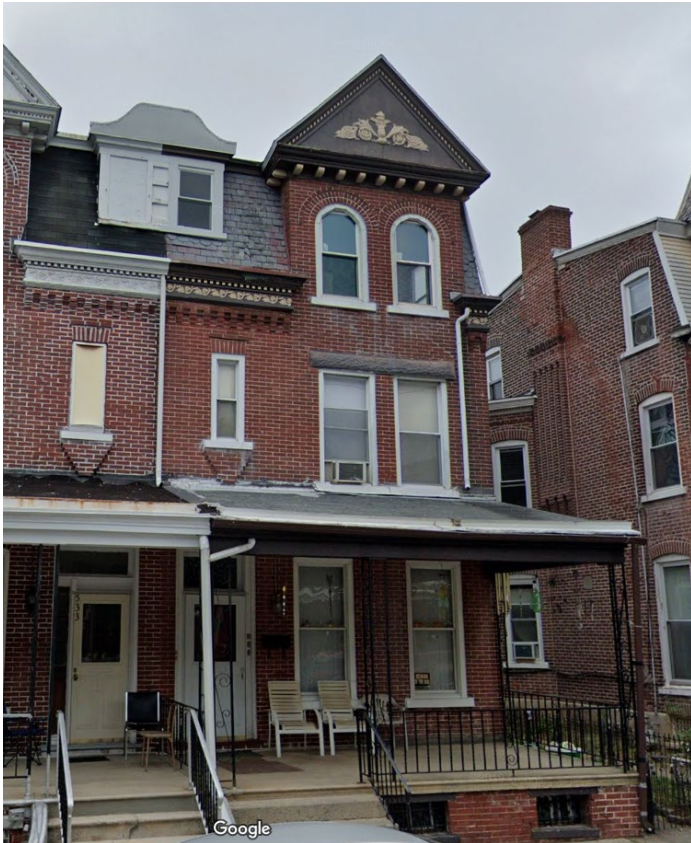
Front façade of 531 W. Allen Street, 2019. (Google StreetView)
