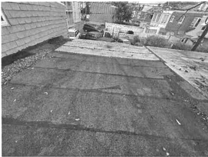
Garage roof -From applicant
