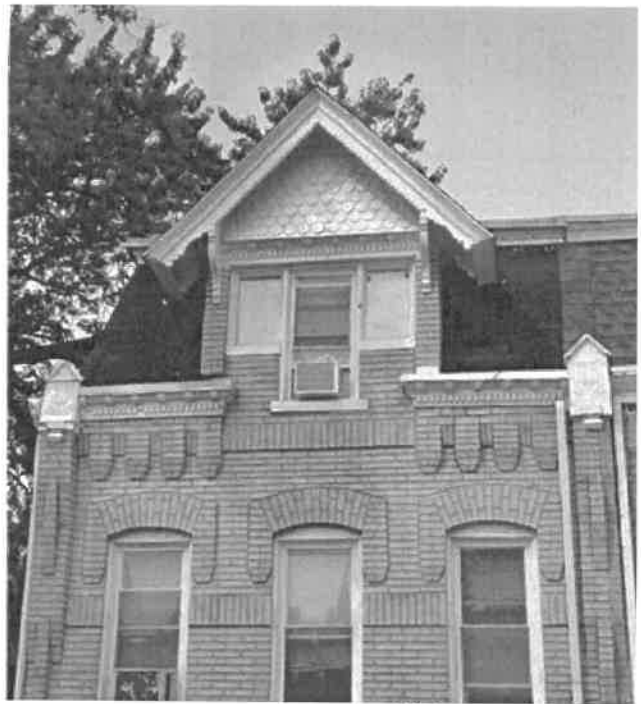
Front windows of 112 N. 11 th Street, current (applicant)
