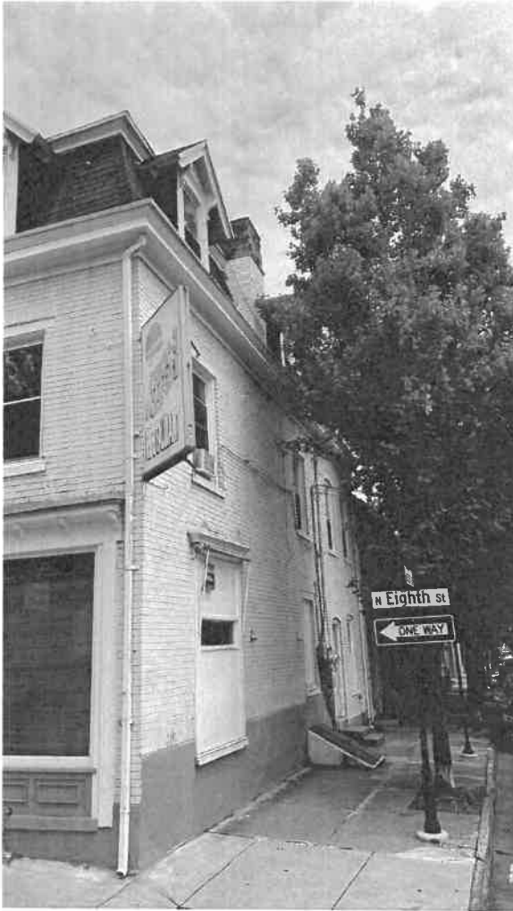
Gordon St facade
