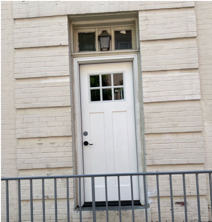
Fiberglass door at Liberty Street façade. (Applicant)
