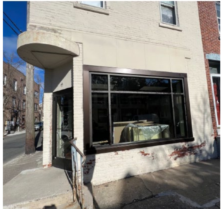
Aluminum storefront window. (Applicant)
