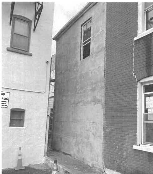
Photo showing rebuilt wall with door moved. (City of Allentown)
