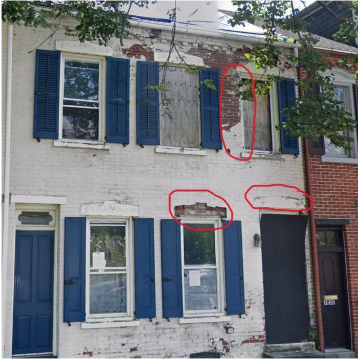
Front Elevation, Missing Window Header (Previous Application)
