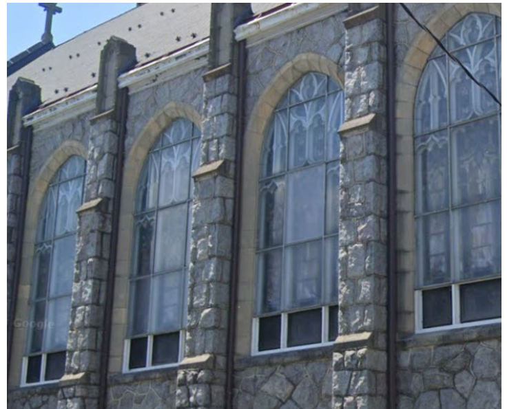
Windows on the east elevation to be replaced, 2023. (Google StreetView)
