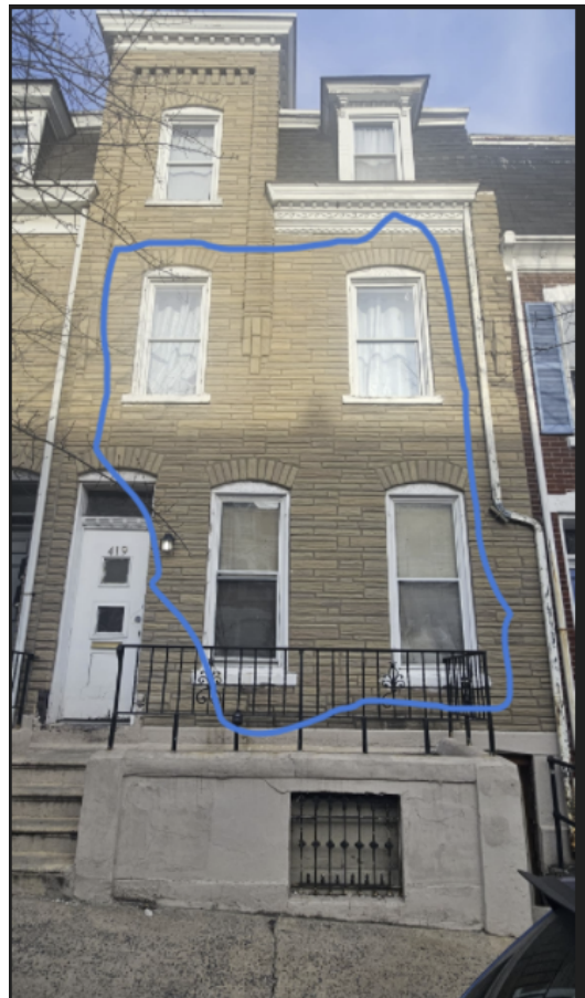
Front windows proposed for replacement (Applicant)
