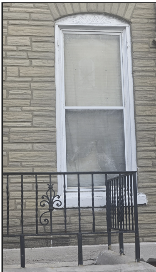
First floor, right side window (Applicant)
