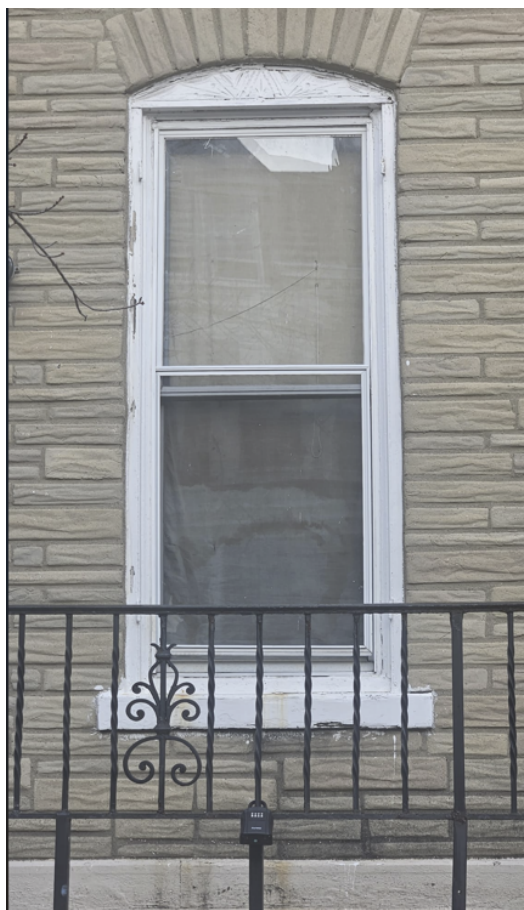
Current first floor, left-side window (Applicant)
