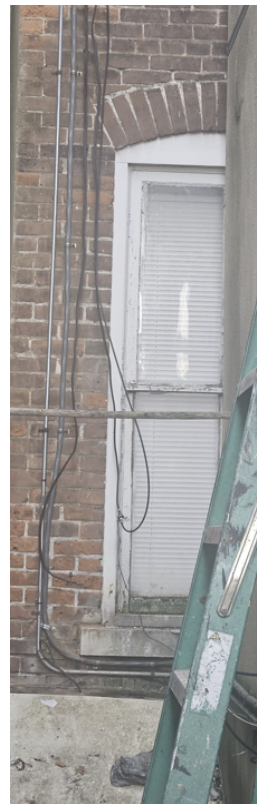
Rear first floor window
