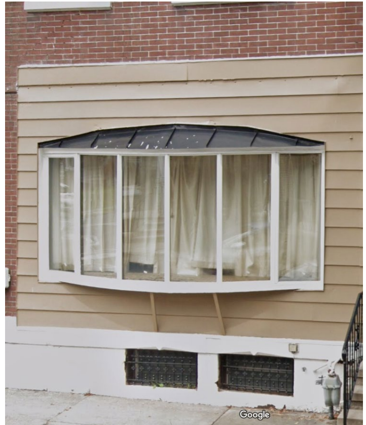
Detail of bow window, 2021. (Google StreetView)
