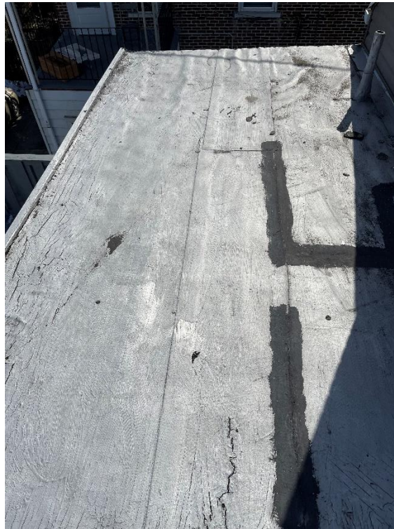
Flat Roof Being Replaced (Applicant)
