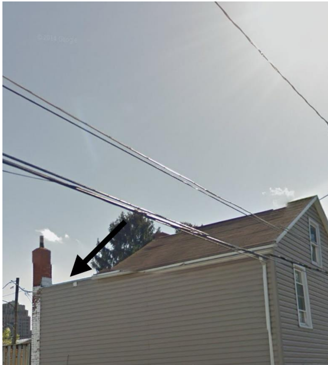
Back of Roof (Applicant)
