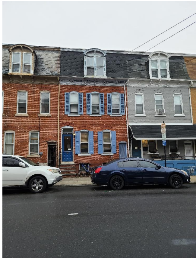
Repaired Roof (Applicant)
