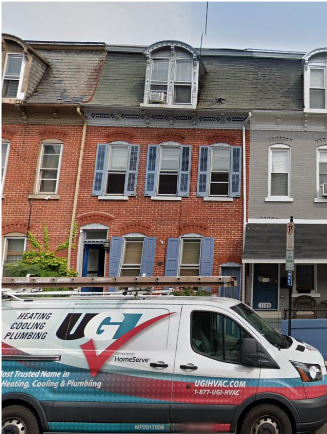
Front Elevation (Google Street View)
