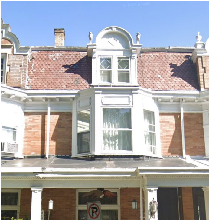
Front roof plane of 1529 Turner Street, 2023. (Google Street View)
