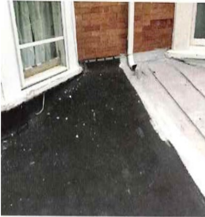
Front porch roof of 1529 Turner Street, 2023. (Applicant)
