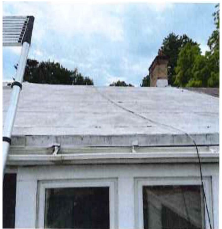
Rear roof plane of 1529 Turner Street, 2023. (Applicant)
