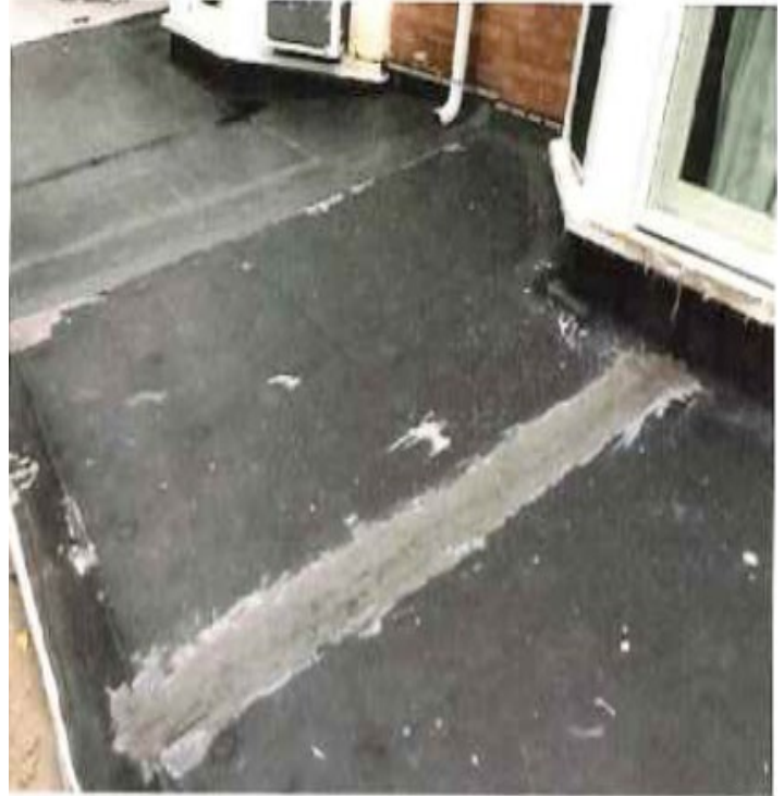
Front porch roof of 1529 Turner Street, 2023. (Applicant)
