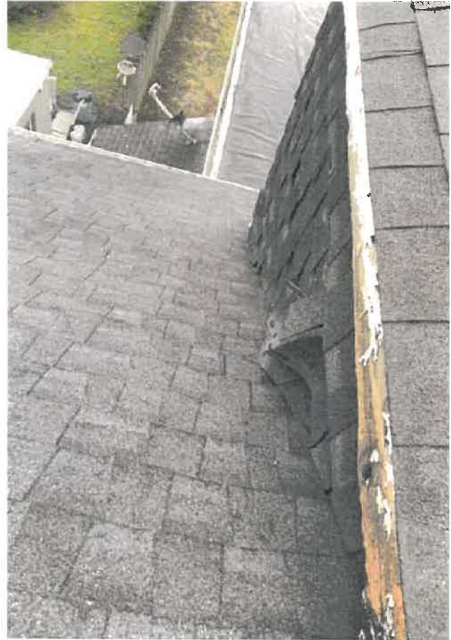
Rear asphalt shingles. (Applicant)
