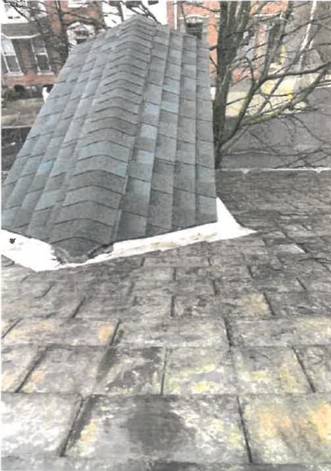
Front slope of roof with original slate (replacement at dormer). (Applicant)
