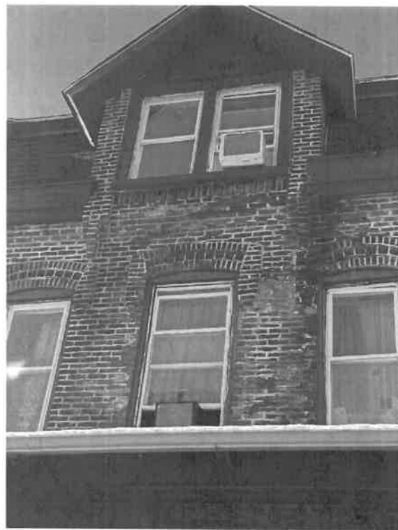
Existing Upper Floor Condition (Applicant)
