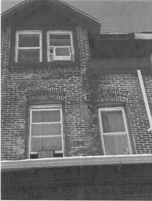
Existing Upper Floor Condition (Applicant)
