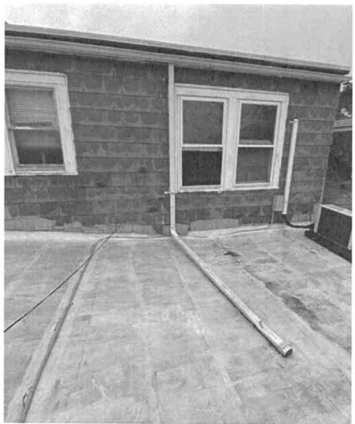
Roof Being Replaced (Applicant)
