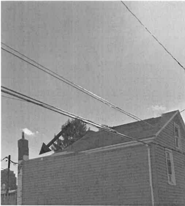
Back of Roof (Applicant)
