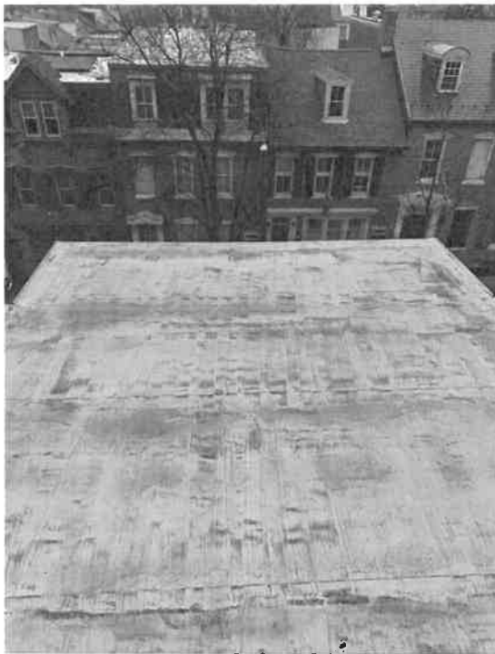
Roof Being Replaced (Applicant)
