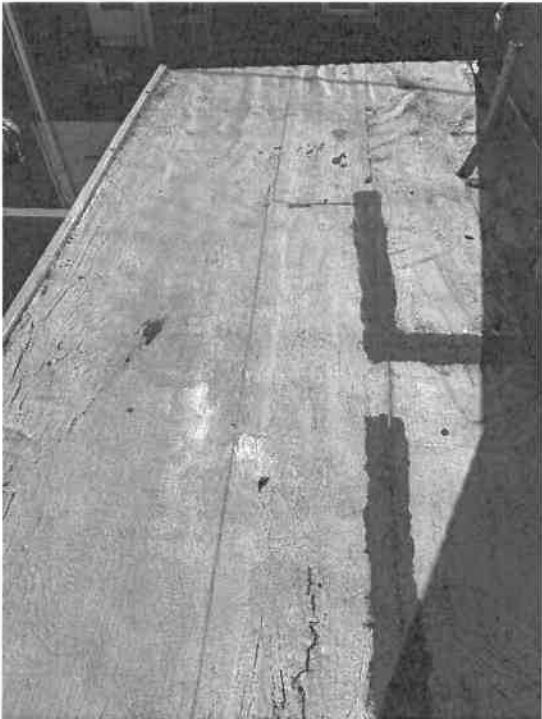
Flat Roof Being Replaced (Applicant)
