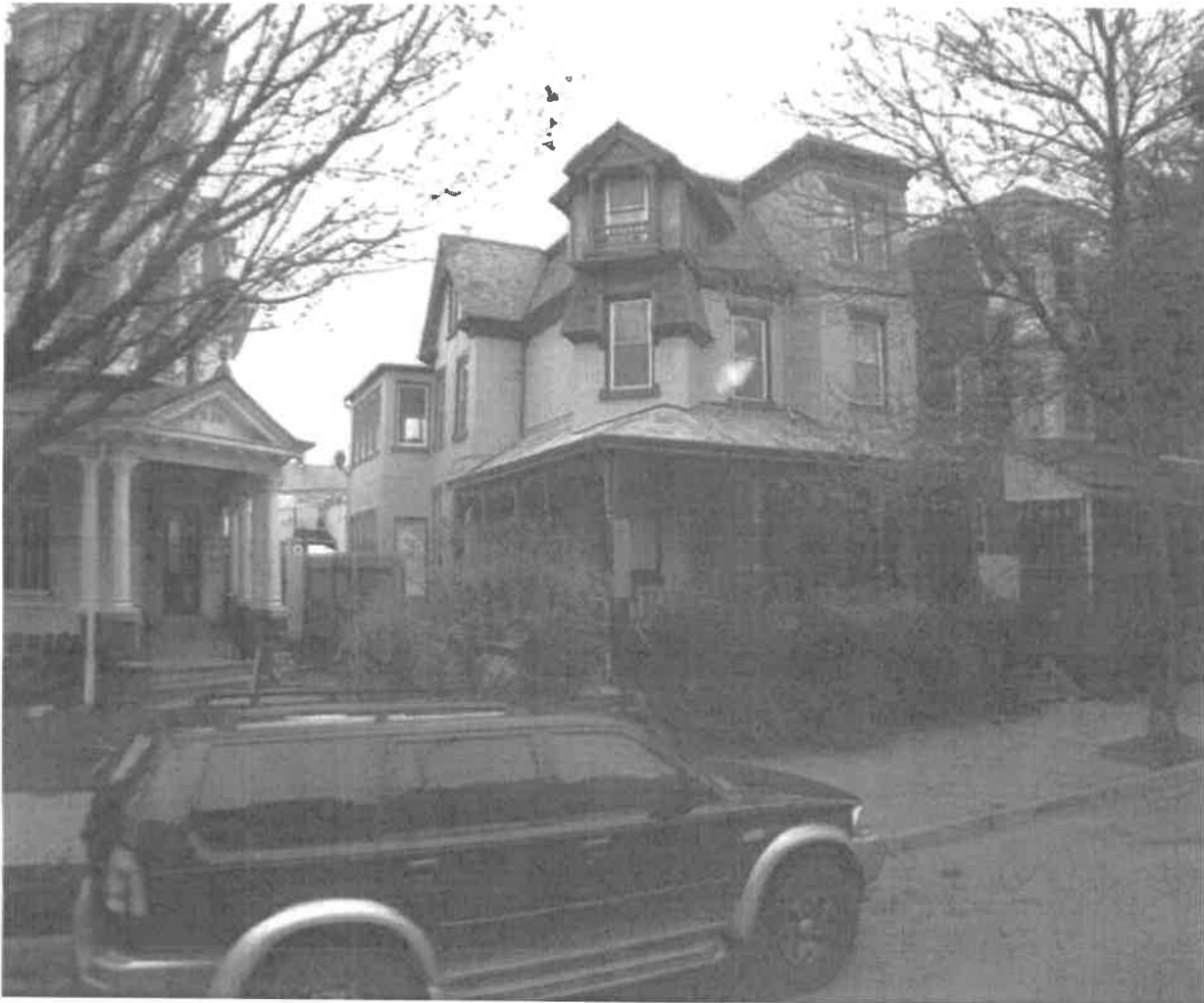
Previous Photograph Prior to Fire Damage (Applicant)
