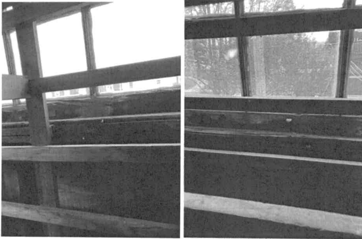
Window Condition (Applicant)
