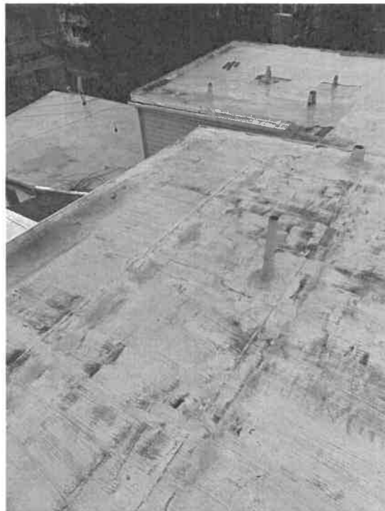
Roof Being Replaced (Applicant)
