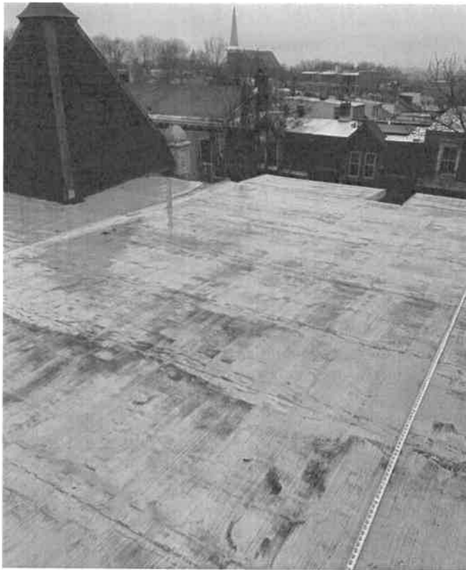
Roof Being Replaced (Applicant)
