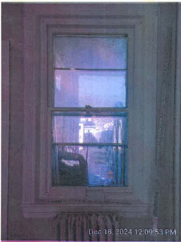
Original Wood Window (Applicant)
