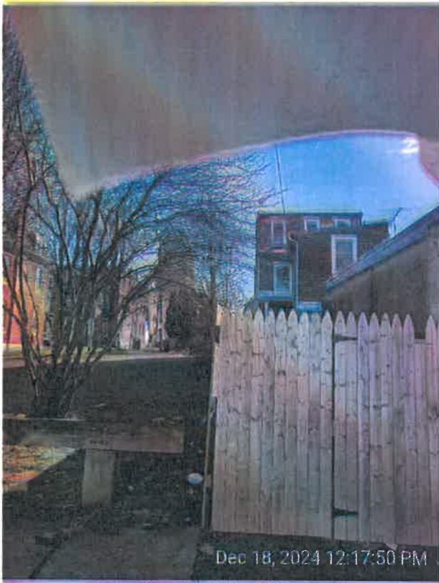
Rear Elevation (City of Allentown)
