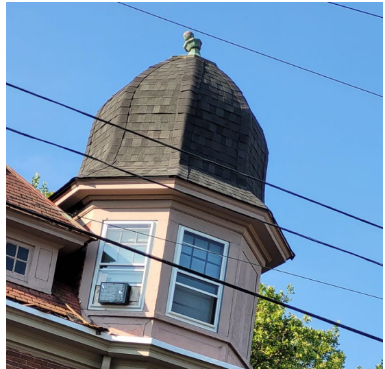
1550-52 W. Chew Street turret roof after work was completed. (Staff)
