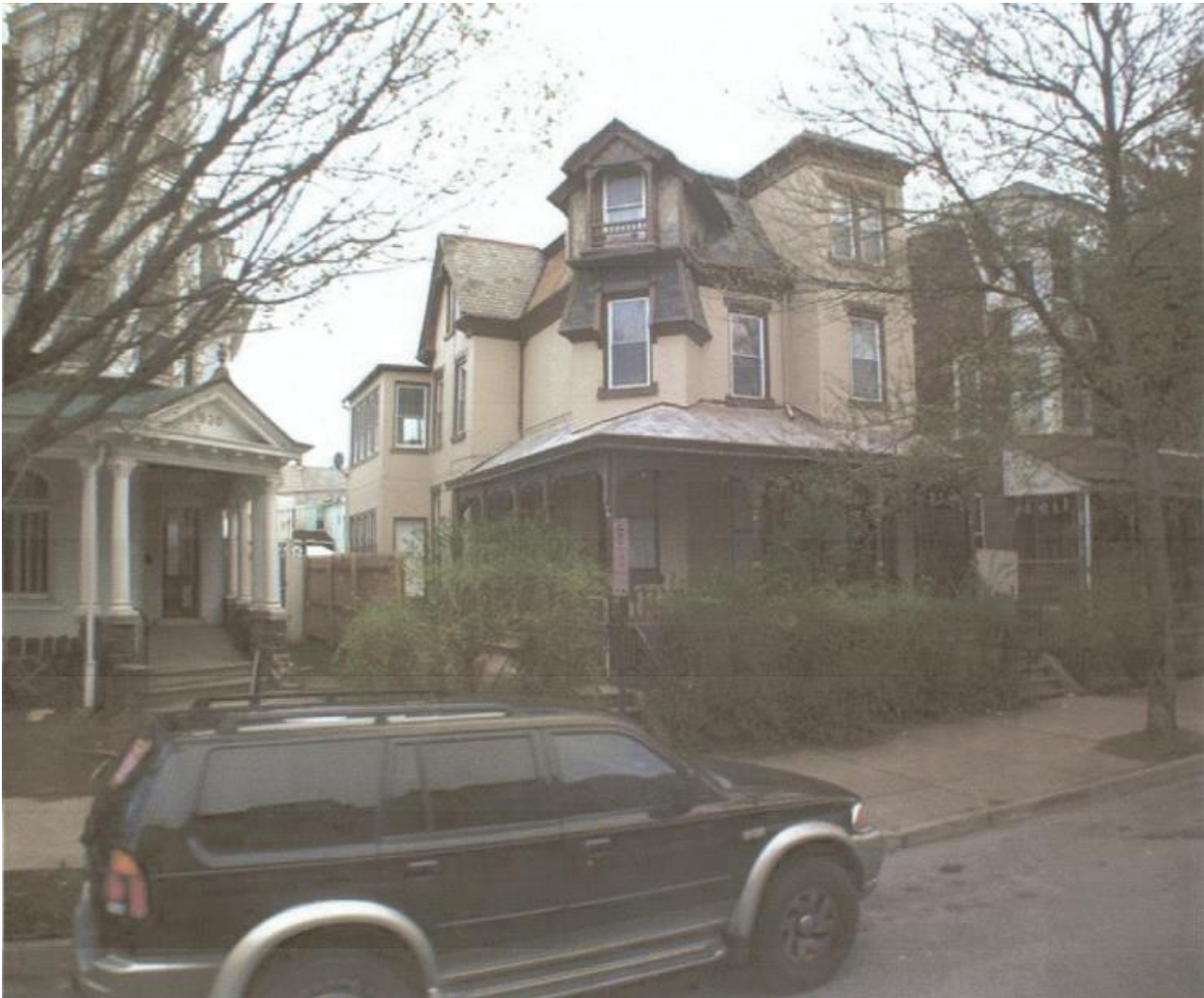
Previous Photograph Prior to Fire Damage (Applicant)
