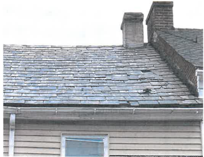
Condition of rear roof, 2023. (Applicant)
