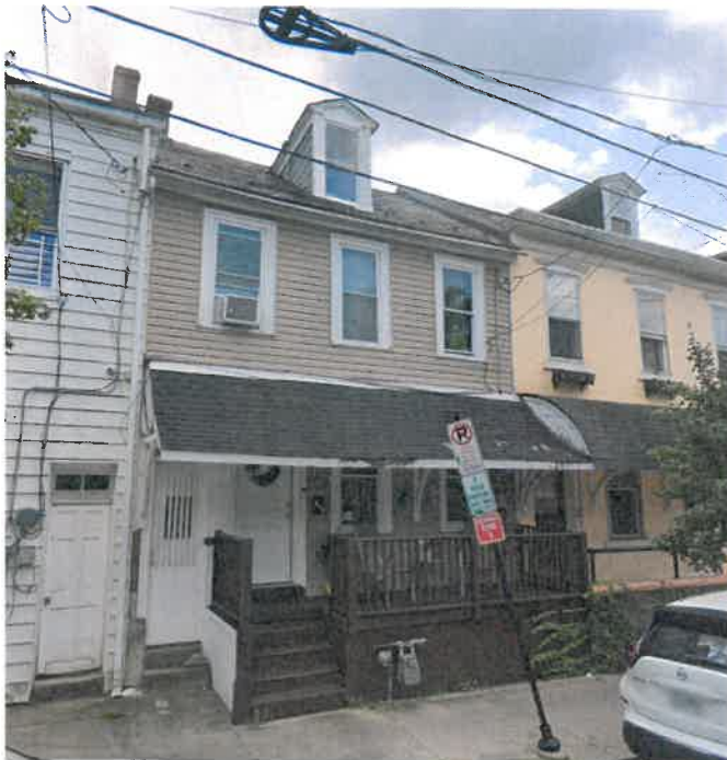
Front façade of 918 W. Chew Street, 2023. (Google StreetView)
