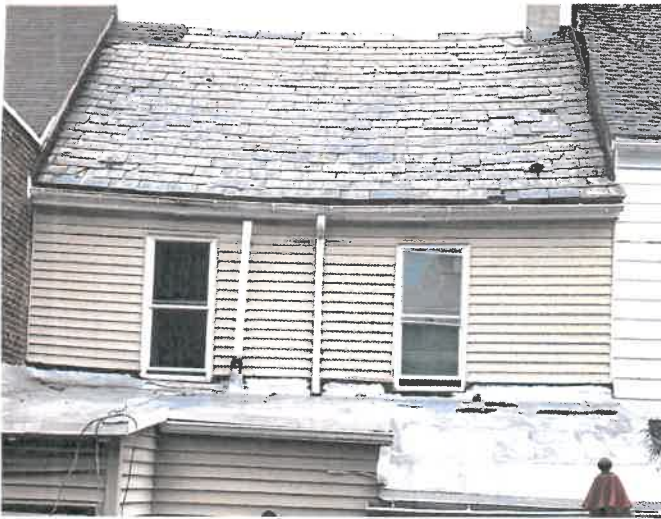
Rear roof of 918 W. Chew Street, 2023. (Applicant)
