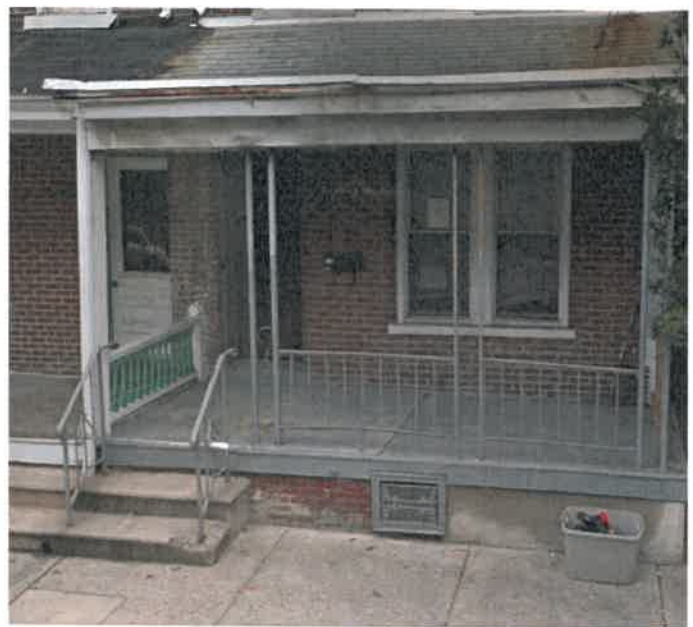
Metal posts and railings prior to replacement, 2018. (Google StreetView)
