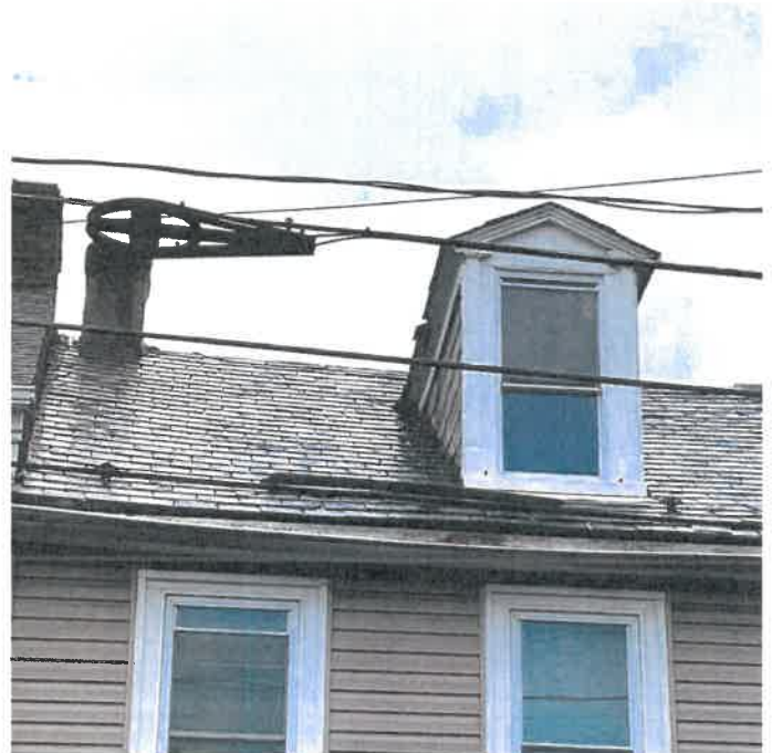
Detail of roof, 2023. (Applicant)
