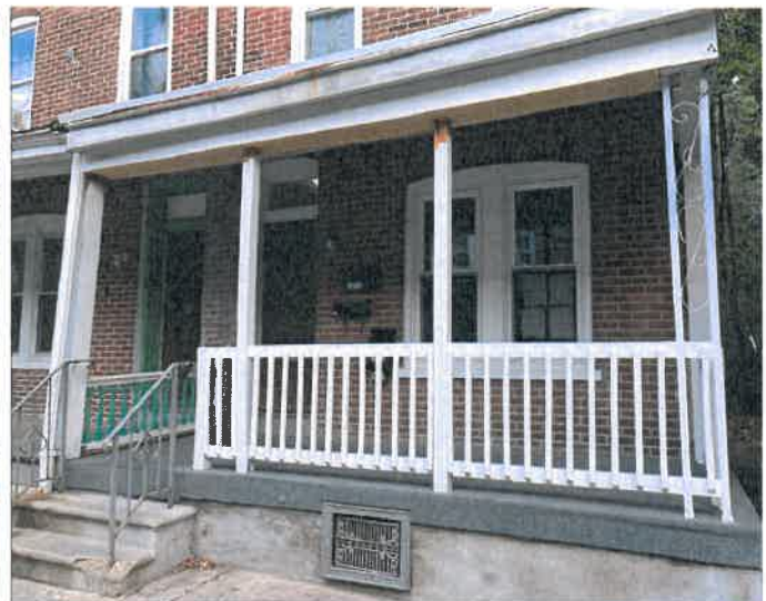
Rear of 141 N. 10 th Street following removal of the porch roof, 2023. (HARB files)
