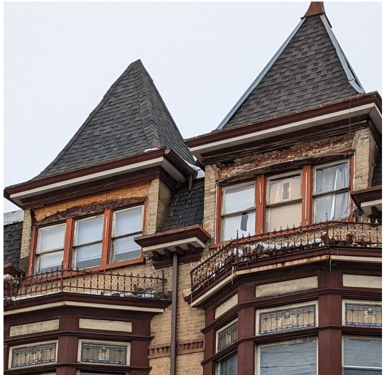
Photo showing the temporary lintel repair at 747 and the fallen brick at the lintel of 745 W. Turner Street, 2022. (HARB files)
