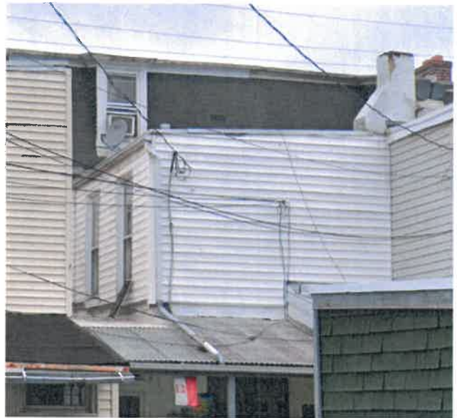
Rear of Property, 2019 (Applicant)
