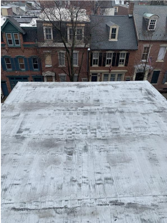
Roof Being Replaced (Applicant)
