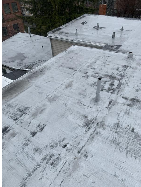
Roof Being Replaced (Applicant)
