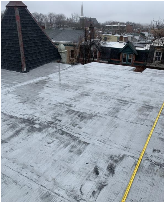
Roof Being Replaced (Applicant)
