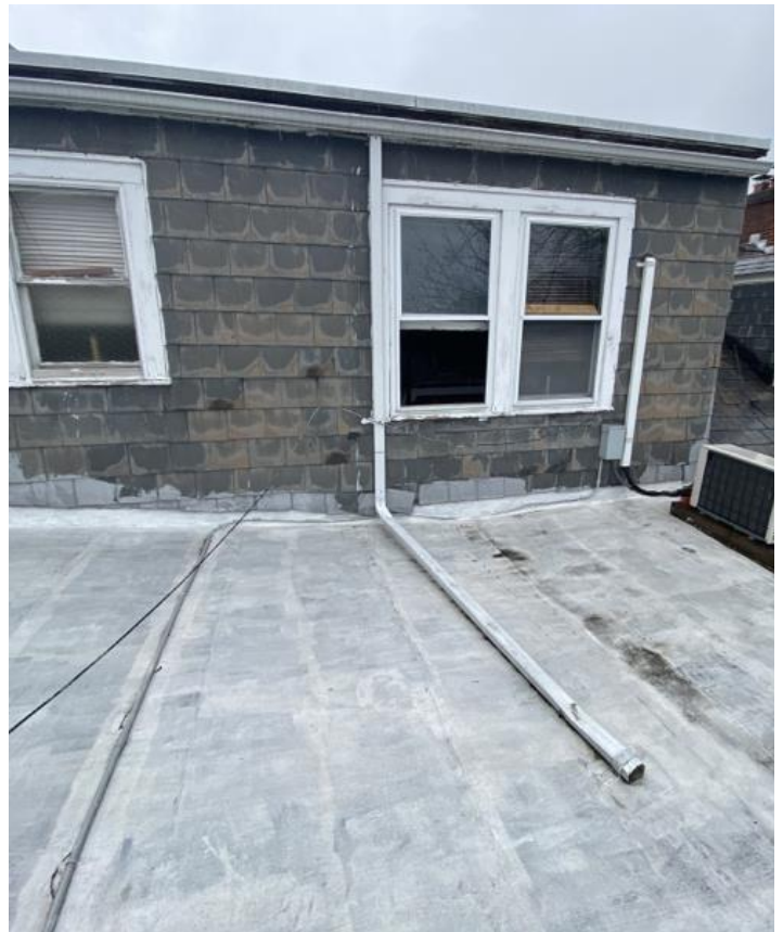
Roof Being Replaced (Applicant)
