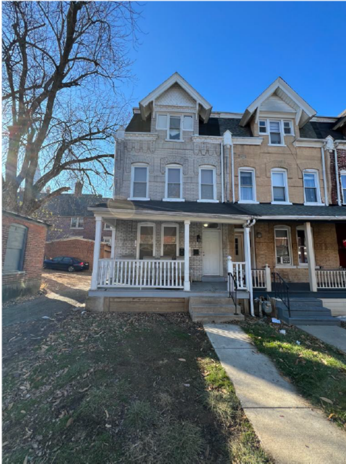
Front facade of 112 N. 11 th Street, current (applicant)
