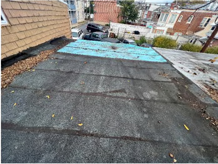
Garage roof -From applicant
