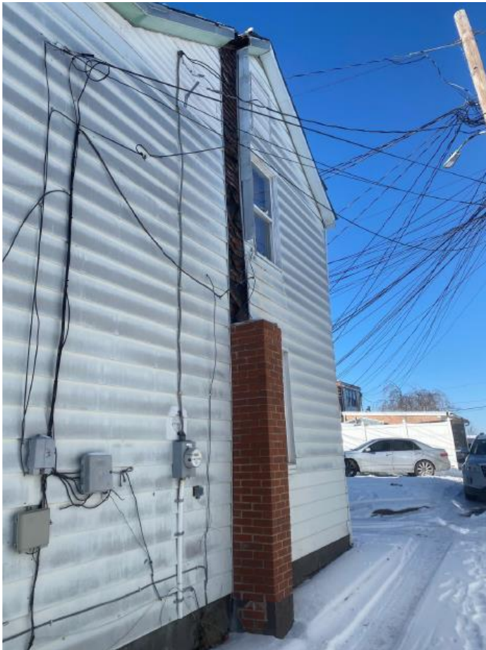
Side facade with chimney at 1142 Emmett Street (applicant)
