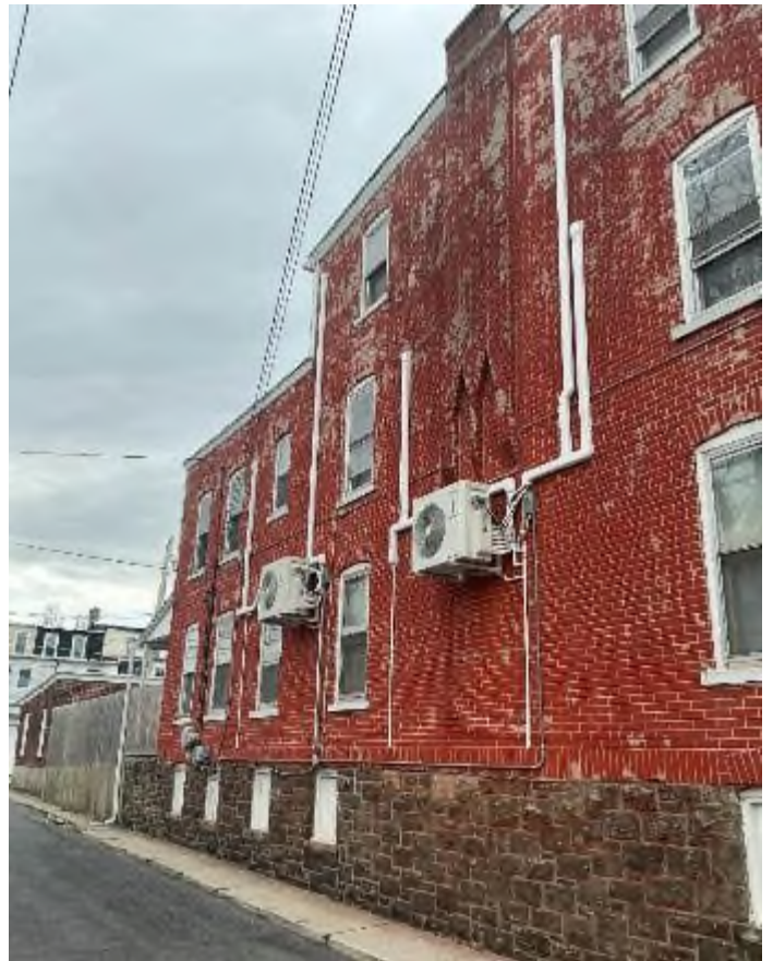
Current Condition, after installation (Applicant)
