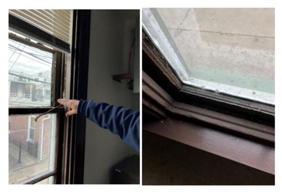
View: West side of building in alley, first floor; window doesn't work, gaps at the bottom, broken pulls.
