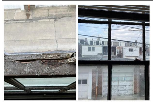
View: West side of the building in alley, first floor; window is damaged, doesn't work. Window Condition (Applicant)
