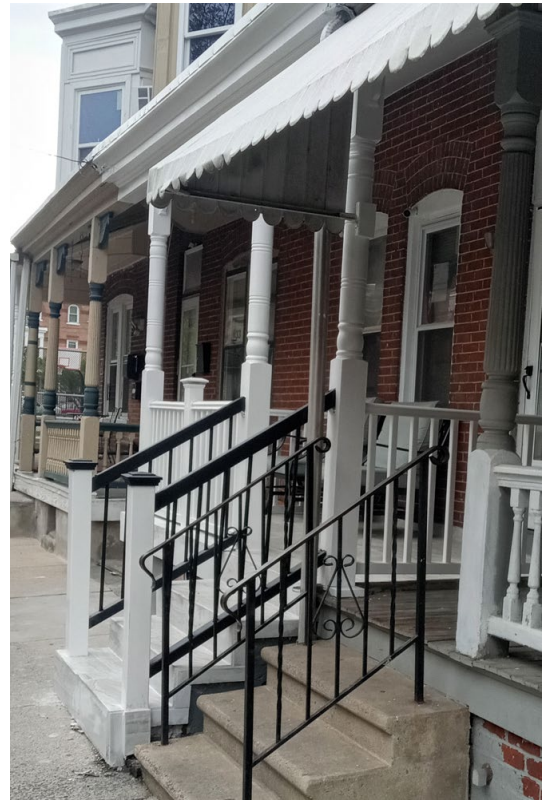
Detail of new railing, 2023. (Applicant)
