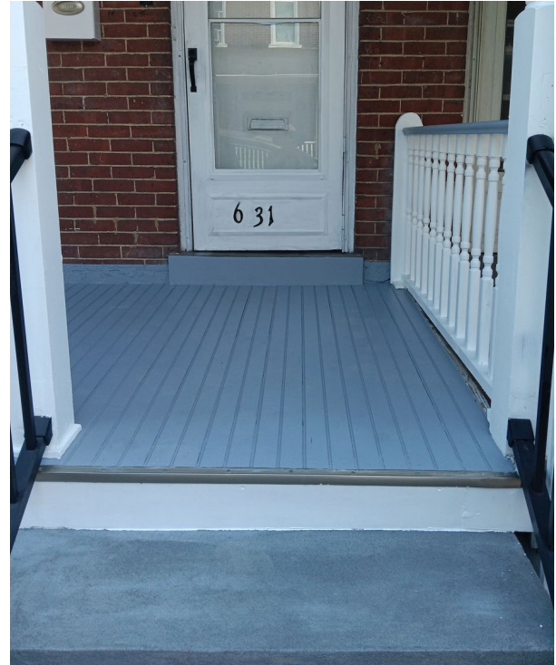
Tongue and groove porch flooring, 2023. (Applicant)
