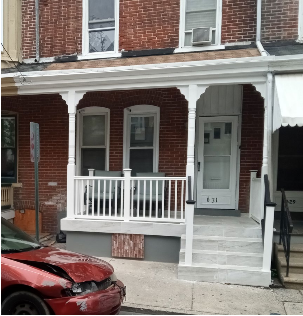
Porch following replacement, 2023. (Applicant)
