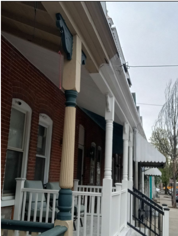
Porch detail following replacement, 2023. (Applicant)
