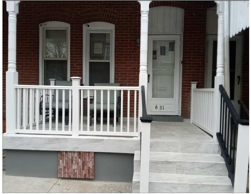
Detail of porch following replacement, 2023. (Applicant)
