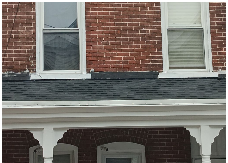
Architectural shingles at porch roof, 2023. (Applicant)
