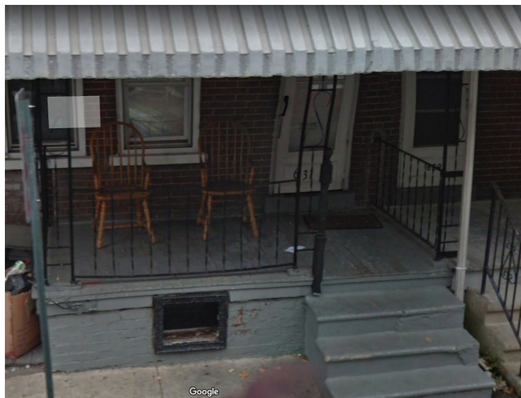
Detail of porch, 2018. (Google StreetView)
