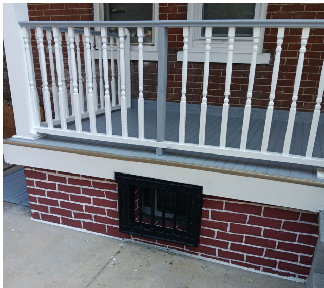
Completed work to correct violation, 2023. (Applicant)
