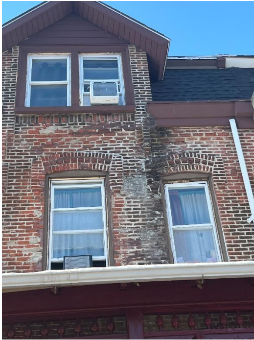
Existing Upper Floor Condition (Applicant)
