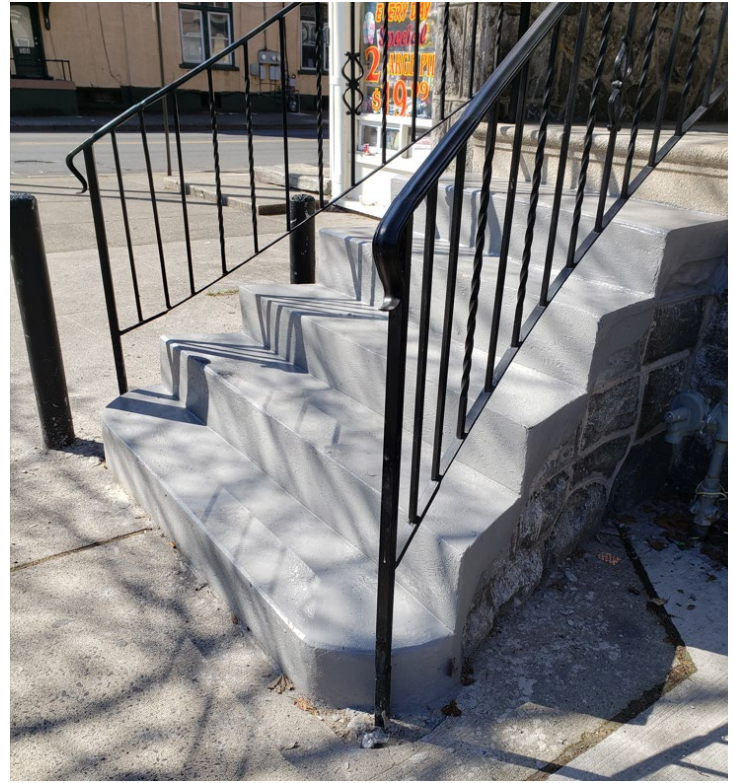
Detail of the stone steps following the cement repair, 2023. (HARB files)
