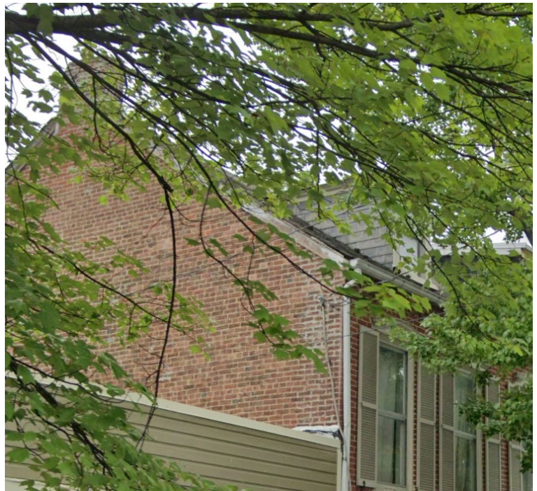
Detail of slate at dormer, 2019. (Google StreetView)
