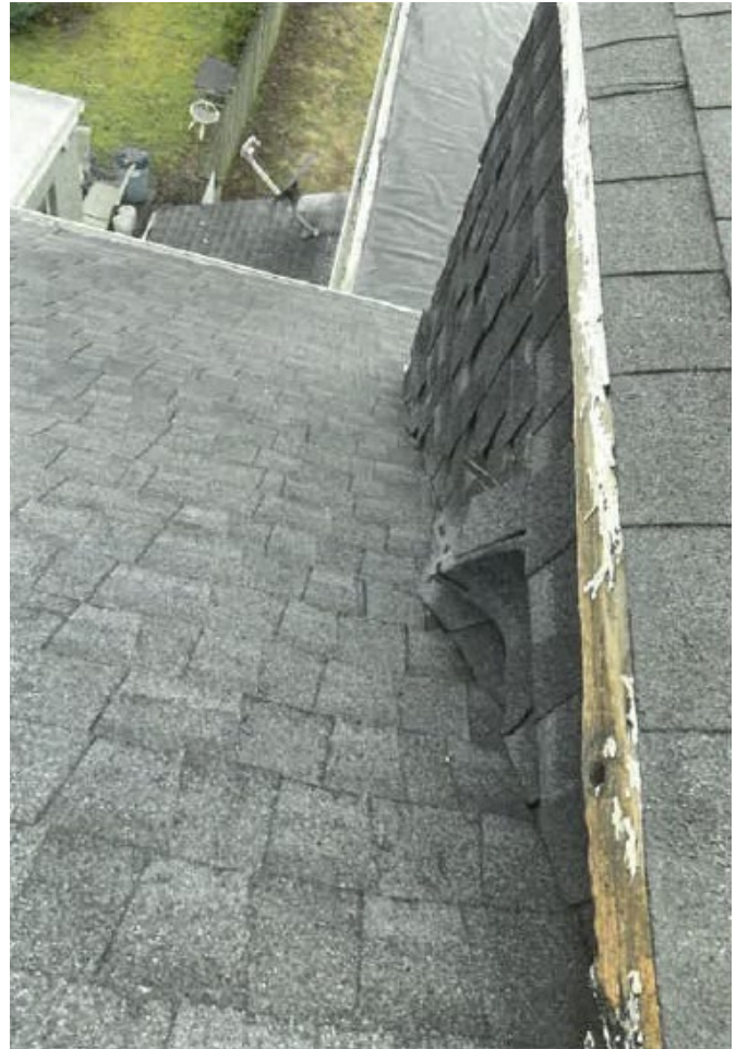
Rear asphalt shingles. (Applicant)
