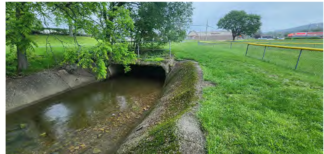
Channelized streams and having lawn up to the edges can create issues with waterways such as introduction of non-point pollutants and flooding when the floodplain has been removed.
