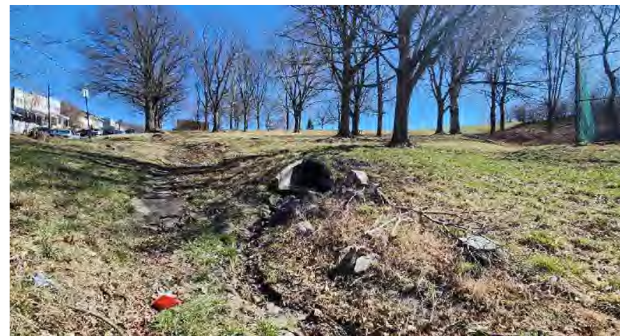
Addressing stormwater in the parks can provide more opportunities for infiltration and filtration of rain water runoff, and address issues caused by channelizing runoff like at Keck Park.
