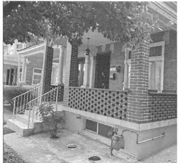
1410 W. Linden Street porch after replacement. (Applicant)
