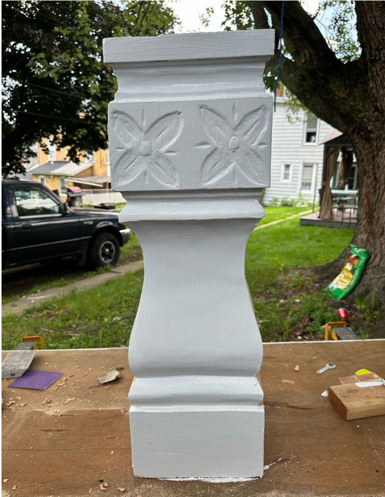
Detail of new column base. (Applicant)
