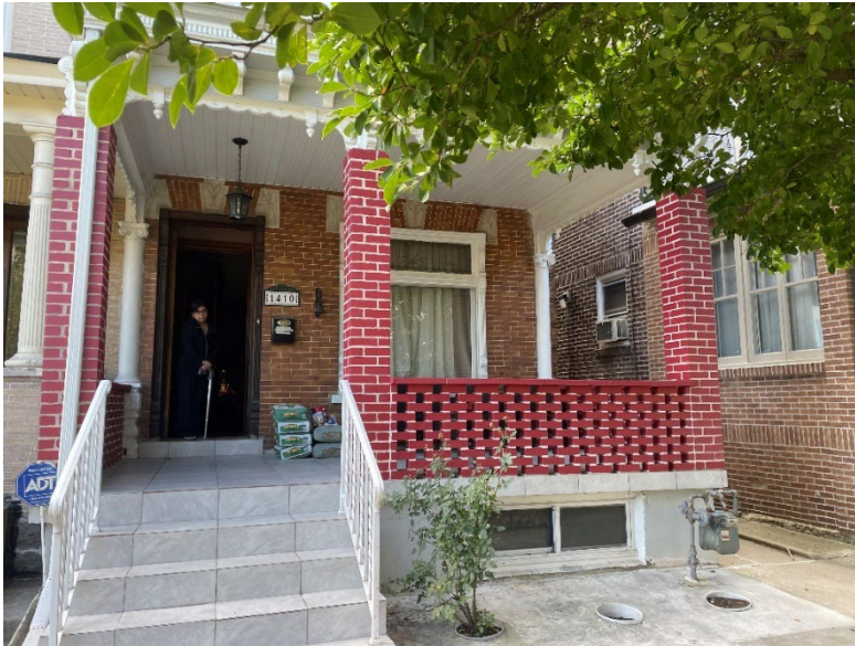
1410 W. Linden Street after replacement. (Applicant)
