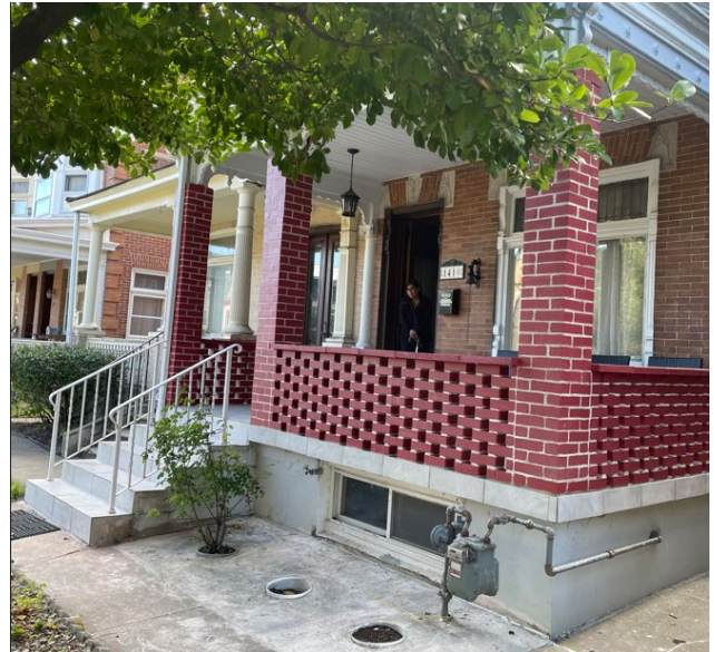
1410 W. Linden Street porch after replacement. (Applicant)
