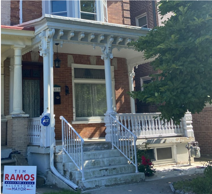
1410 W. Linden Street porch prior to replacement, 2021. (Easton Architects)
