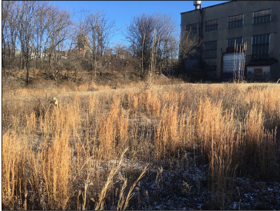
Photo 15. A view of the building on the northern edge of the northernmost project area.
