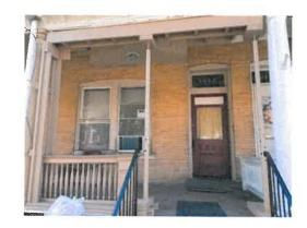
Proposed alterations: It is proposed to repair the porch columns, header, and wall.
