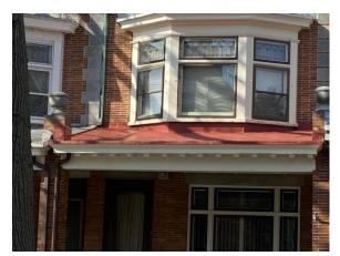
**Proposed alterations:** It is proposed to replace red tin porch roof with black rubber roofing material.
