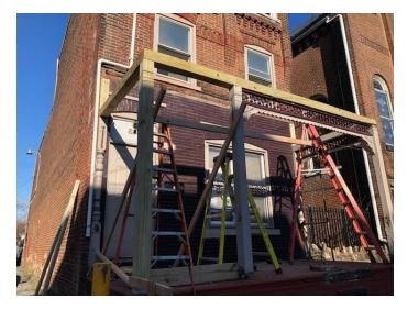
Proposed alterations: It is proposed to rebuild porch and repair/replace the turret roof.
