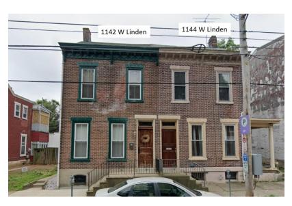
**Proposed alterations:** It is proposed to install a fence and repair brick façade. The wooden fence will be extended to the front property line using the same 6' high dog ears design wooden fence. The exterior façade brickote will be stripped, any damaged brick repaired and repointed.
