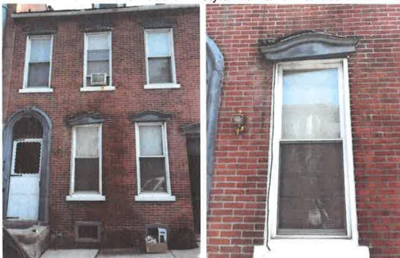
**Proposed alterations:** It is proposed to replace deteriorated original lintels and other wood trim with Fypon to match original as close as possible.
