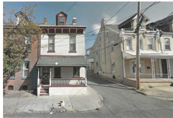
Allentown, Pennsylvania Google, Inc. Street View - Oct 2014
