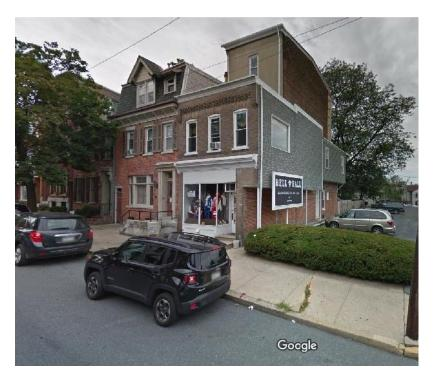
**Proposed alterations:** It is proposed to continue installation of vinyl siding over insulating siding, commonly known as Insul-Brick, on the side of the building and to install vinyl siding along the remainder of the side of the building currently covered with similar insulating siding. **Staff Approvals:** N/A
