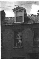
**Proposed alterations:** It is proposed to replace the deteriorated slate roof with Heritage Premium laminated asphalt shingles in Virginia Slate color.
