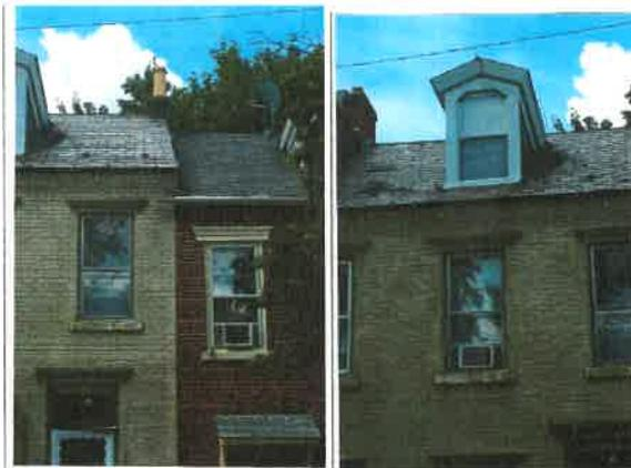
**Proposed alterations:** It is proposed to replace the deteriorated slate roof with Heritage Premium laminated asphalt shingles in Virginia Slate color.
