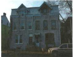
**Proposed alterations:** It is proposed to modify the previous COA on brickote. The existing brickote will be repaired, stained in brick red color and joints pointed on the front façade to create a more authentic brick look.
