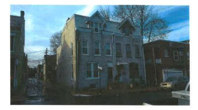
**Proposed alterations:** It is proposed to modify the previous COA on brickote. The existing brickote will be repaired, stained in brick red color and joints pointed on the front façade to create a more authentic brick look.
