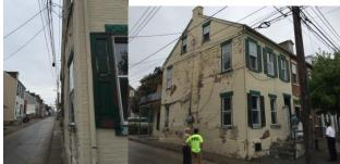
**Proposed alterations:** It is proposed to demolish the building. The brick east wall is in poor condition and has a bulge. Interior inspection revealed floor joists coming out of packets due to the outward movement of the wall. The building is owned by a mortgage servicing company and appears to have been a foreclosure in 2015. The building is currently vacant.
