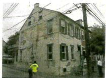
**Proposed alterations:** It is proposed to demolish the building. The brick east wall is in poor condition and has a bulge. Interior inspection revealed floor joists coming out of packets due to the outward movement of the wall. The building is owned by a mortgage servicing company and appears to have been a foreclosure in 2015. The building is currently vacant. **Staff Approvals:** n/a
