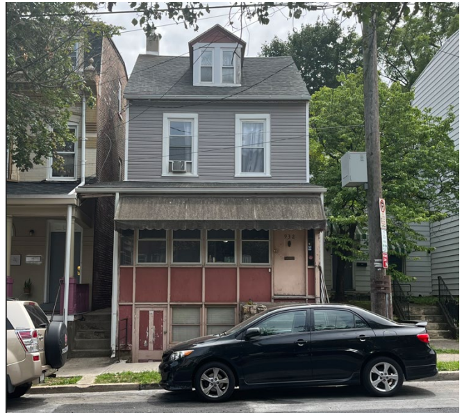
Front façade of 932 W. Gordon Street after work, 2023. (Applicant)
