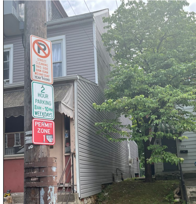
Side façade after siding was installed, 2023. (applicant)
