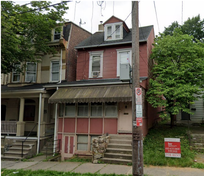
Front façade of 932 W. Gordon Street, 2019 (Google StreetView)
