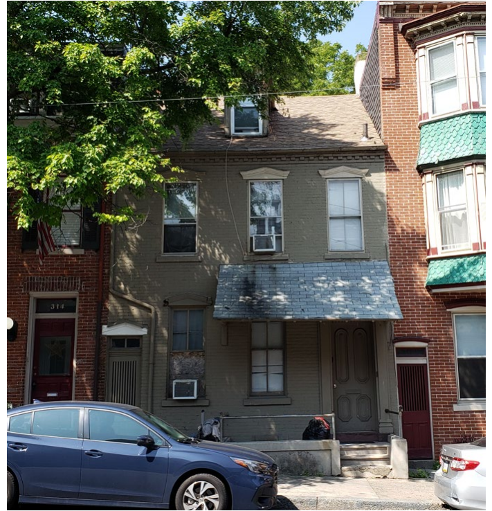
Back Roof Aerial of 213 N. 11 th Street, 2023. (HARB files)
