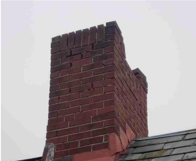
Current Chimney (Applicant)
