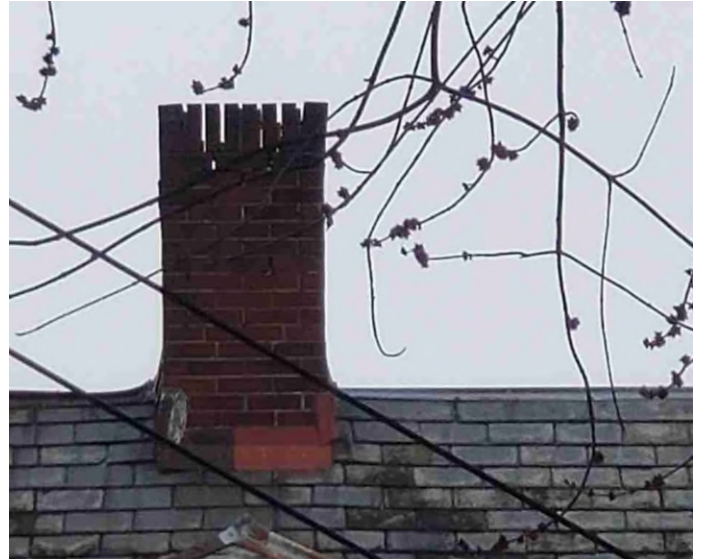
Current Chimney (Applicant)
