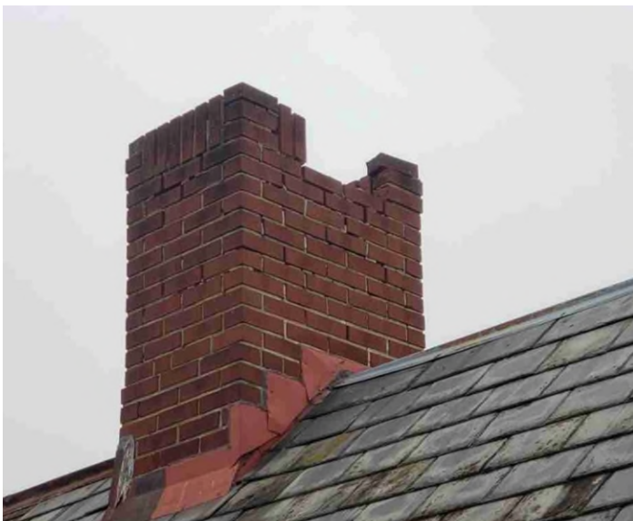
Current Chimney (Applicant)
