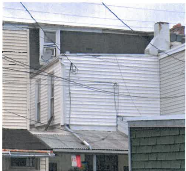
Rear of Property, 2019 (Applicant)
